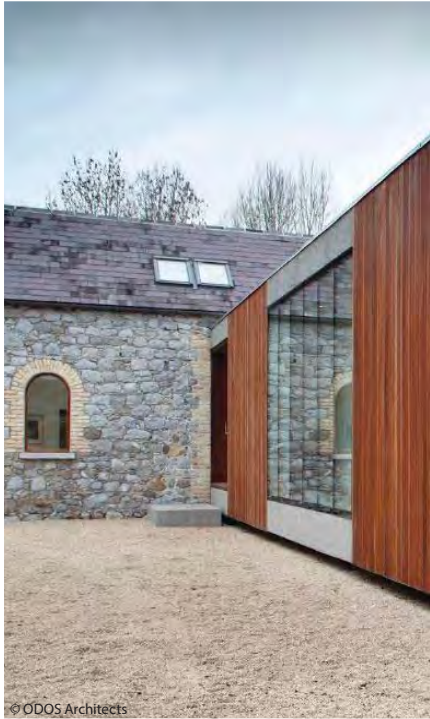
© ODOS Architects Ballymahon, by ODOS Architects
